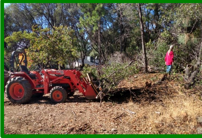
Removing dense brush at house next to Oak Hill Rd
