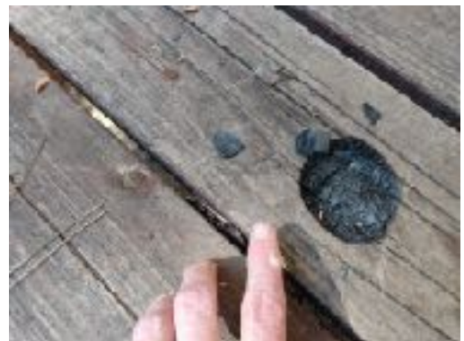
Ember Char on deck. Returning evacuees were thankful that pine needles were recently removed and that their deck was clear of anything flammable.
